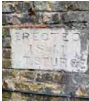
Existing historic plaque retained and re-purpose into a concrete wall
