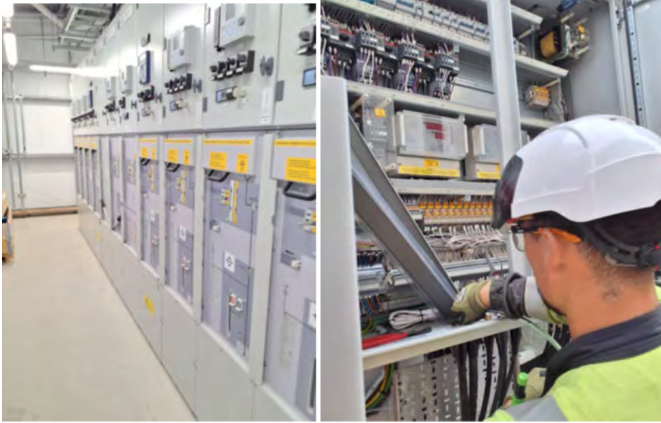
11kV switchboard wiring and cold commissioning
