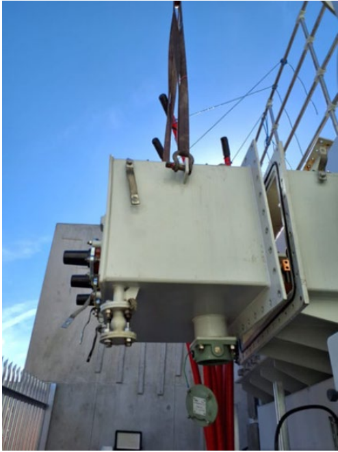
Figure 2. Transformer cable tail installation.
