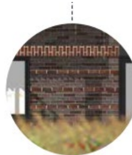
Red brick soldier course separating the base from the levels above with dark rusticated brickwork at base
