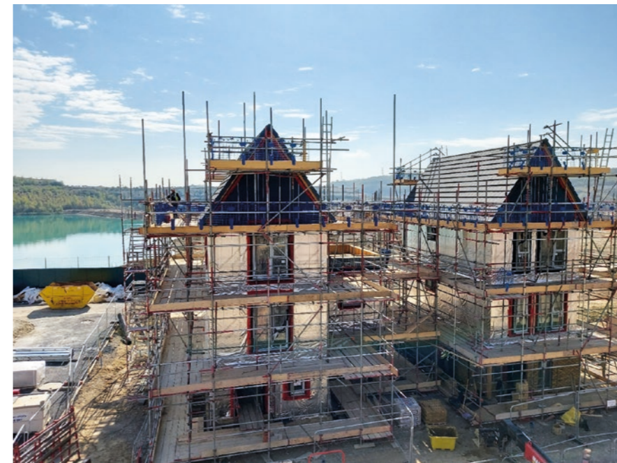
Figure 3: Western Cross (Ashmere) Phase 1 under construction.
