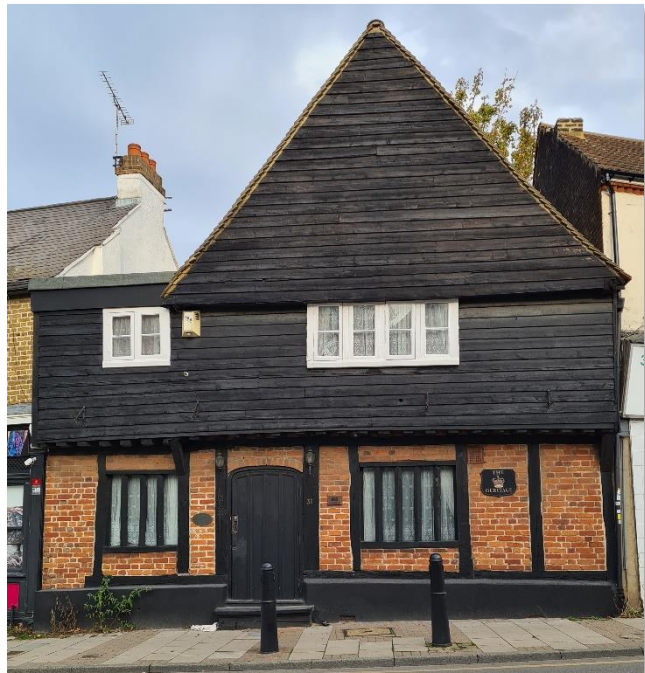
Figure 5.10: Medieval building (31 the Hill) opposite church of St Botolph, Northfleet
